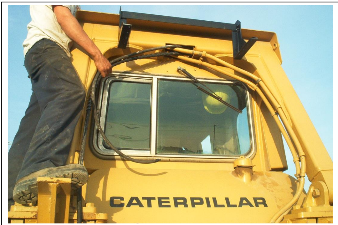
Hoses coming out for condenser.
