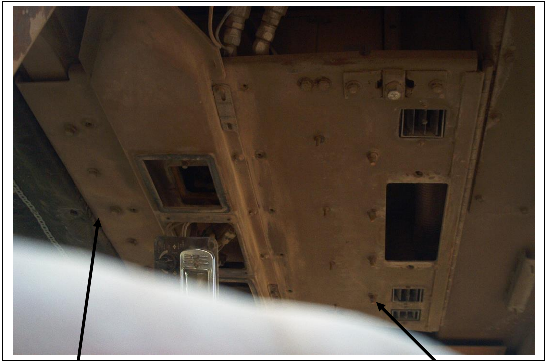
Removed these 5 bolts
