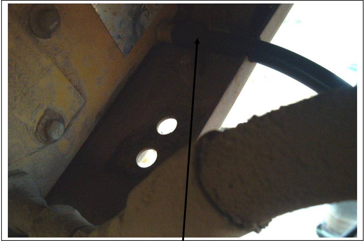
Drain tube installed.
